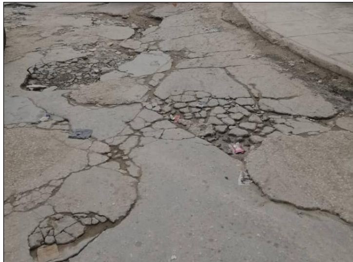
Figure 11: Shows the situation of the asphalt in one of the side roads (roads within residential areas).
